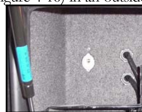
Figure 4-16. Cable & Telephone Jack
