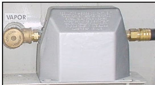
Figure 3-5. LP Gas Regulator
