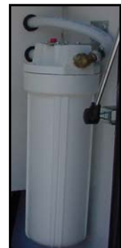
Figure 11-8. Water Filter
