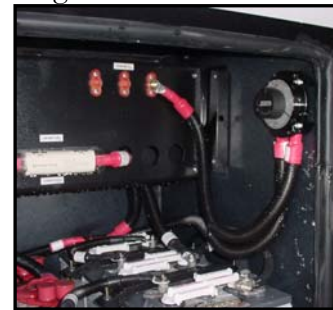
Figure 7-7. House Battery Disconnect Switch (right side)
