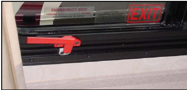
Figure 13-2. Bedroom Emergency Exit Window
