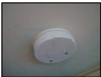
Figure 2-7. Smoke Detector
