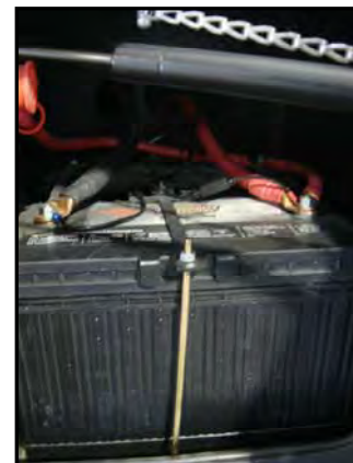
Figure 7-5. House Batteries (Underneath Entrance Door Step Well)
