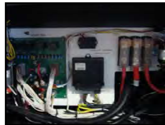
Figure 7-4. 12 VDC Battery System
