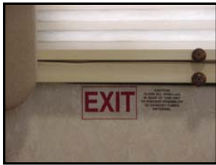
Figure 13-2. Emergency Exit Window
