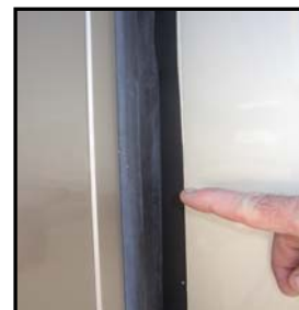
Figure 14-5. Inspecting Slide Out Gasket
