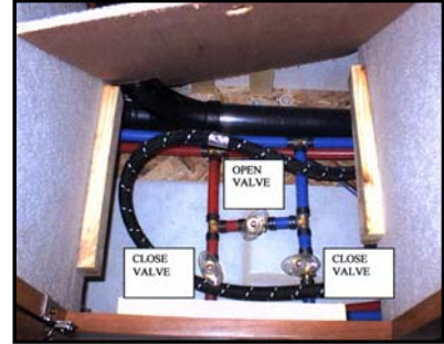
Figure 11-8. Water Heater Bypass System
