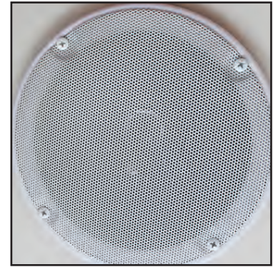
Figure 6-3: Overhead surround sound speaker
