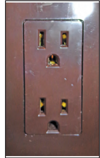
Figure 9-2: 120 VAC receptacle
