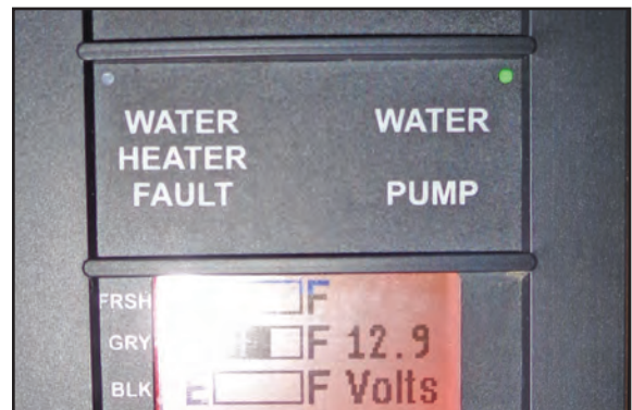
Figure 13-5: Water pump switch
