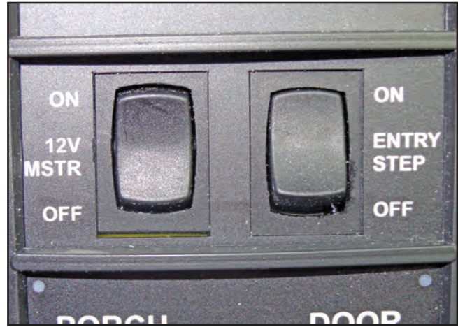
Figure 9-12: 12 VDC disconnect switch
