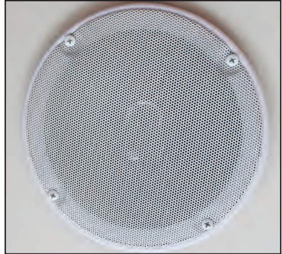
Figure 6-3: Overhead surround sound speaker
