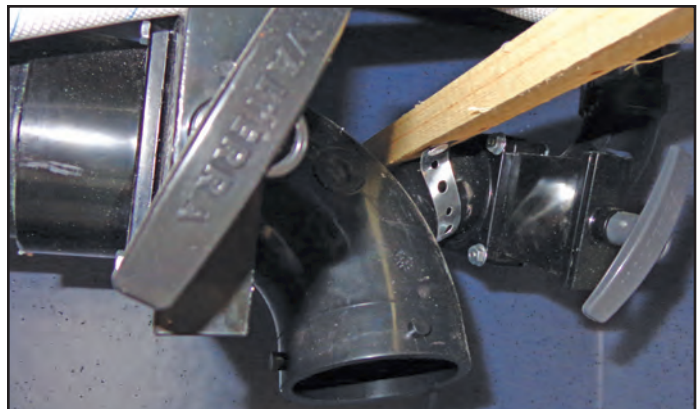
Figure 13-11: Sanitation coupling, valve and hose
