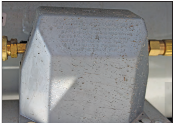
Figure 4-2: LP Gas Regulator
