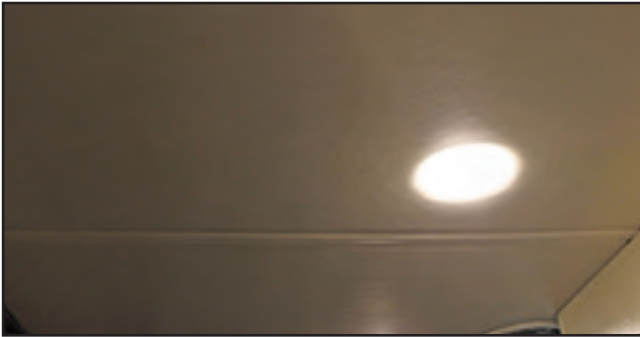
Figure 12-3: Typical ceiling in the Allegro
