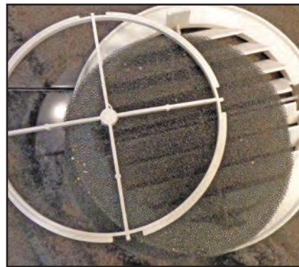
Figure 3-3: Round vent filter
